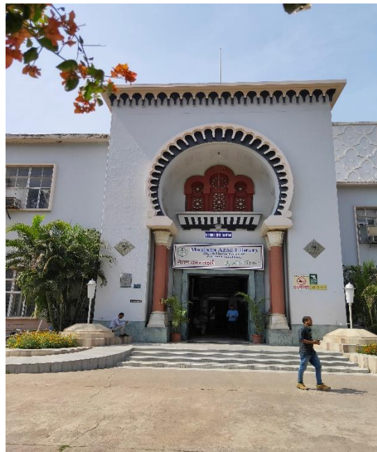
Figure 2.2: Maulana Azad Library (Main entrance)
